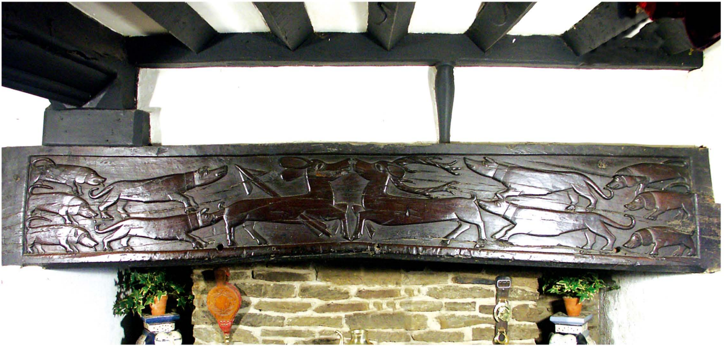
265 (above) Fireplace beam, oak. Lower Spoad, Clun, Shropshire. Tree-ring dated to 1546.
